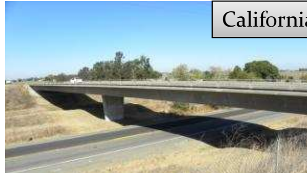
2-span prestressed post-tensioned continuous CIP box girder
